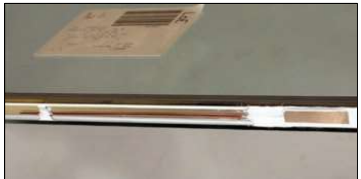
Fig 2 An installed capillary tube, colored red for photo only
