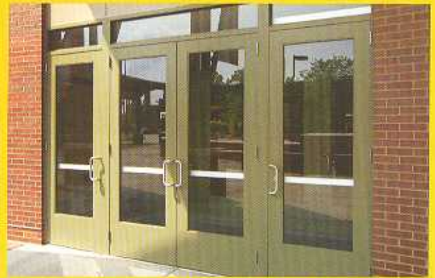
Custom Entrance, Green Painted Finish; Project: Andrews Student Recreation & Wellness Center, Youngstown State University, Youngstown, OH; Architects: Strollo & Associates; General Contractor: Hively Construction; Tubelite Dealer: Warren Glass
