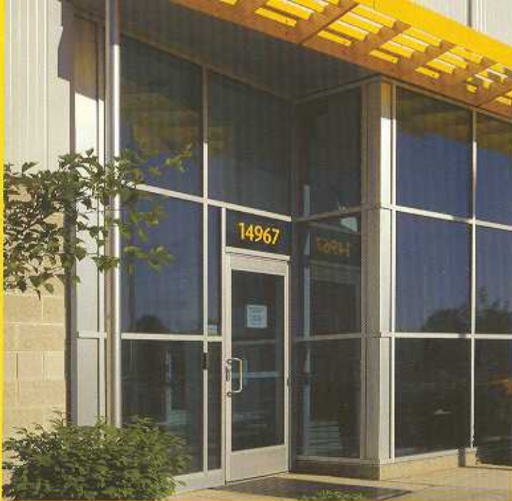
Custom Entrance, Clear Anodized; Owner: Karmann Manufacturing, Plymouth, MI; Architect: DeMottia Group; Tubelite Dealer: Calvin & Company
