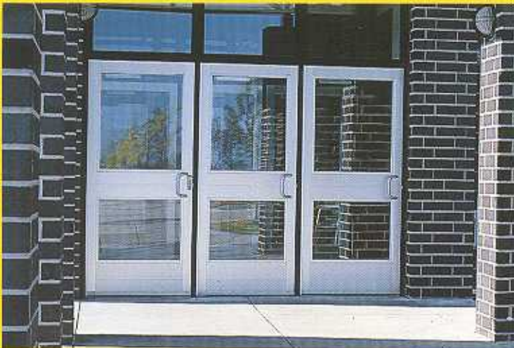
Custom Entrance, 3K Clear Anodized; Big Rapids High School, Big Rapids, Michigan; Architect: GMB Architects; Tubelite Dealer: Valley Glass
