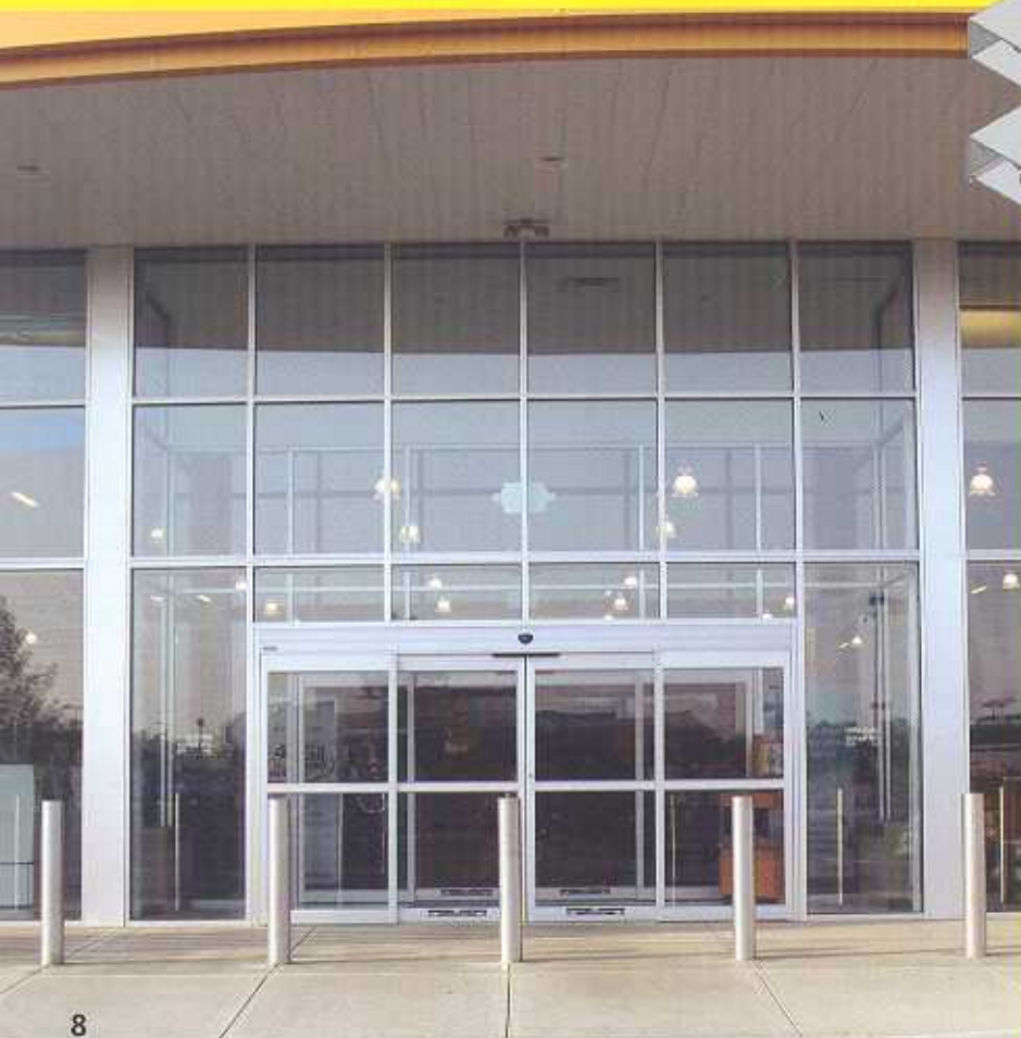
14650 Series Storefront, 0A Clear Anodized; Owner: HH Gregg/Fine Lines Appliances, Columbus, OH; Architect: Herschman; General Contractor: Corna Kokosing; Tubelite Dealer: Richardson Glass
